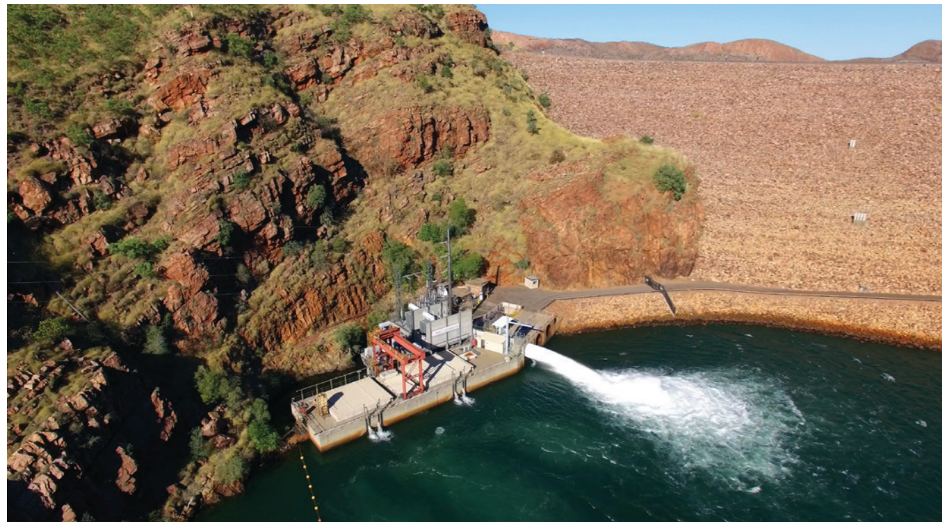
ABOVE: Ord Hydro Plant, Western Australia
