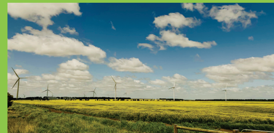
ABOVE: Yaloak South Wind Farm, Victoria
