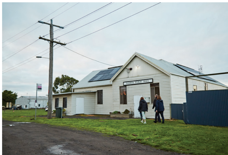
TOP: Anthony Leddin and his family walking to the Yambuk Public Hall BOTTOM: The Yambuk Public Hall proudly displaying the new solar system provided by Pacific Hydro
