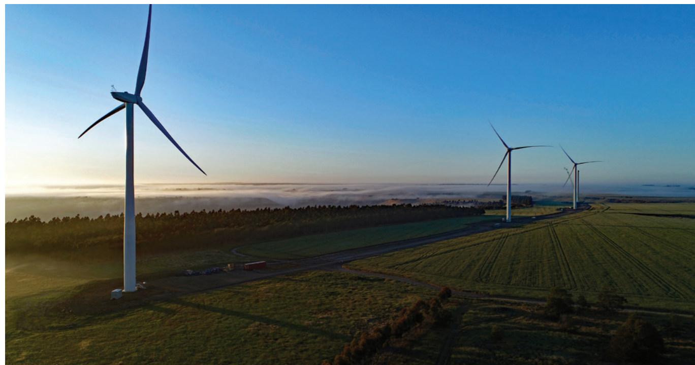
ABOVE: Yaloak South Wind Farm, Victoria
