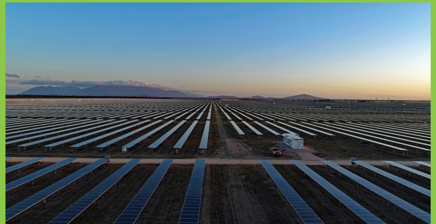
ABOVE: Houghton Solar Farm, Queensland
